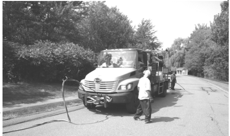
Sealing of the cracks in the roadways and driveways by New England Sealcoating.
